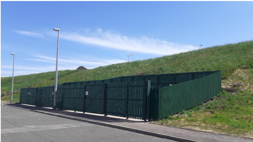
Waste compound on Gunsgreen Quay
